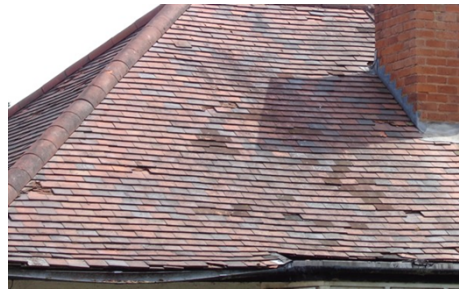
missing roof tiles allowing water to penetrate
