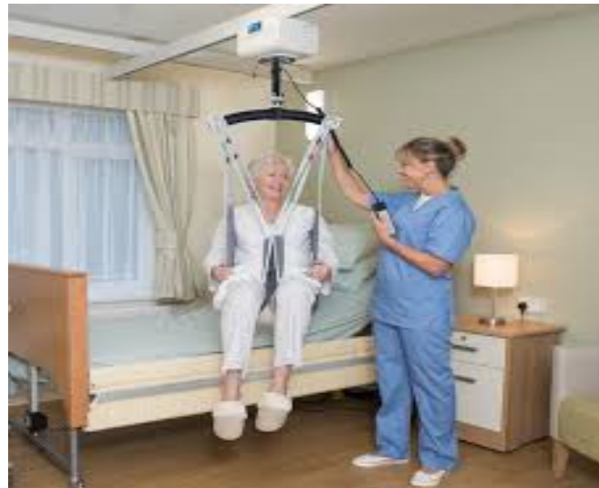
Hoists (Ceiling Track)
