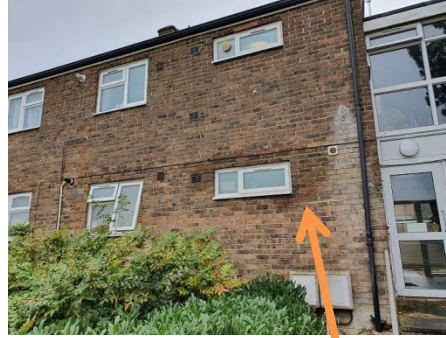
Visible wet area externally
